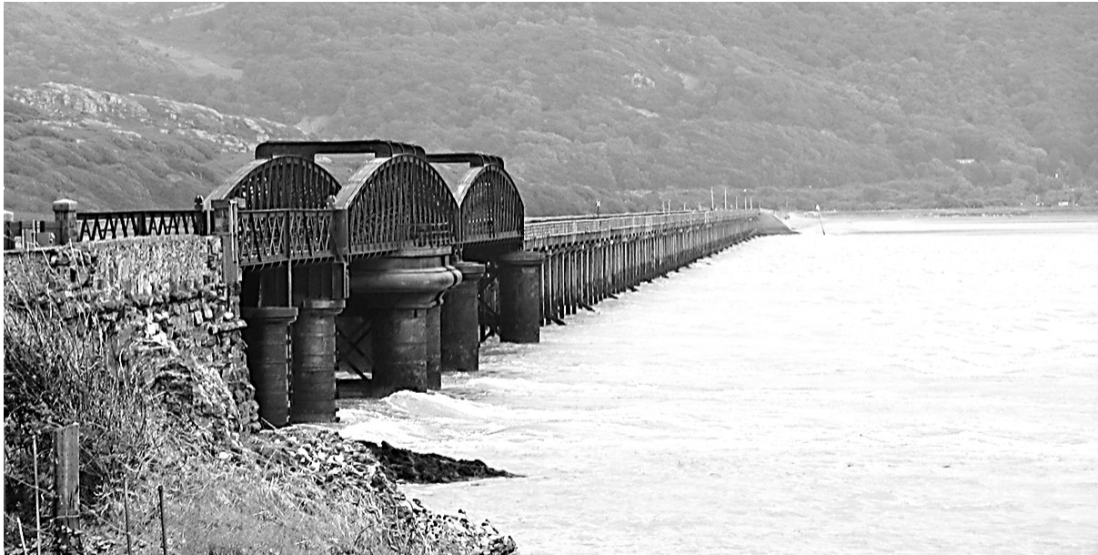
Figure 230: Barmouth railway viaduct at the mouth of the Mawddach estuary
